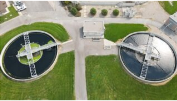
North and South Clarifiers
