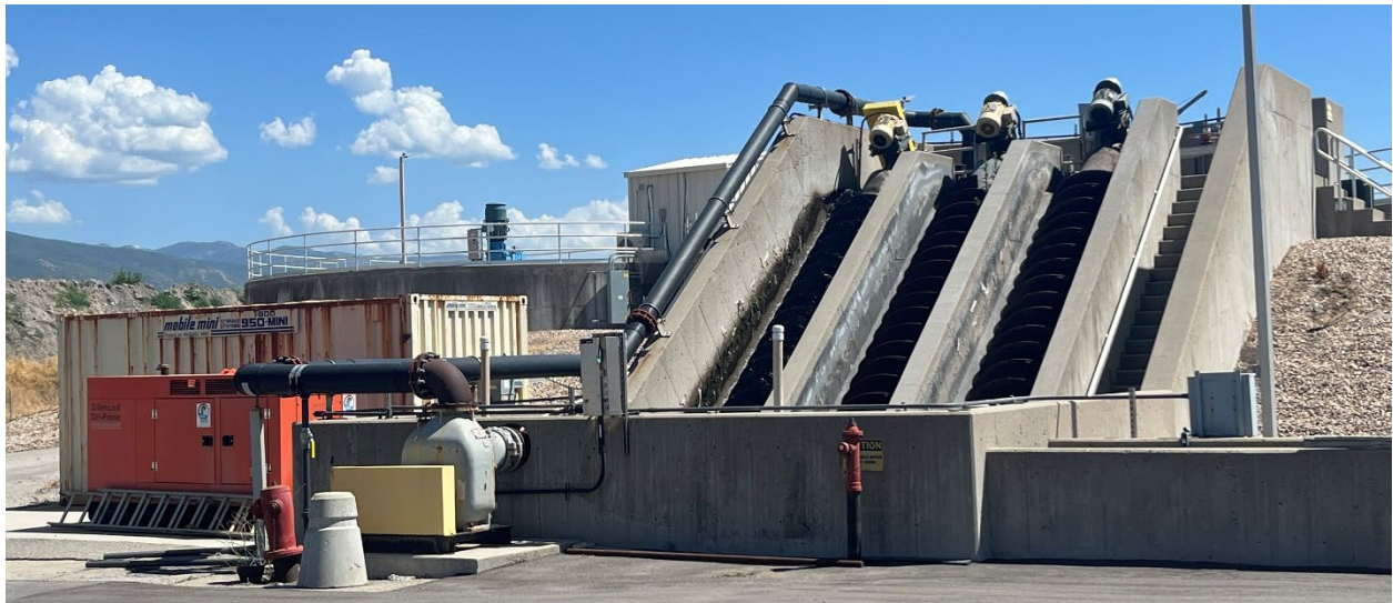
Figure 7: Screw Pump Station and Generators
