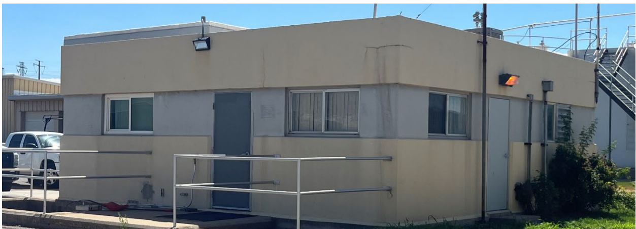
Figure 20: Trickling Filter Primary Pump Station Building
