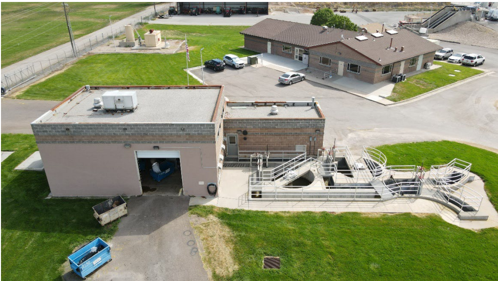
Figures 2: Headworks Arial Photos
