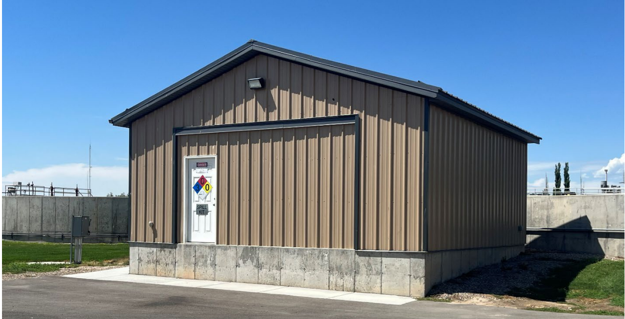
Figure 9: Oxidation Ditch Alum Building and System
