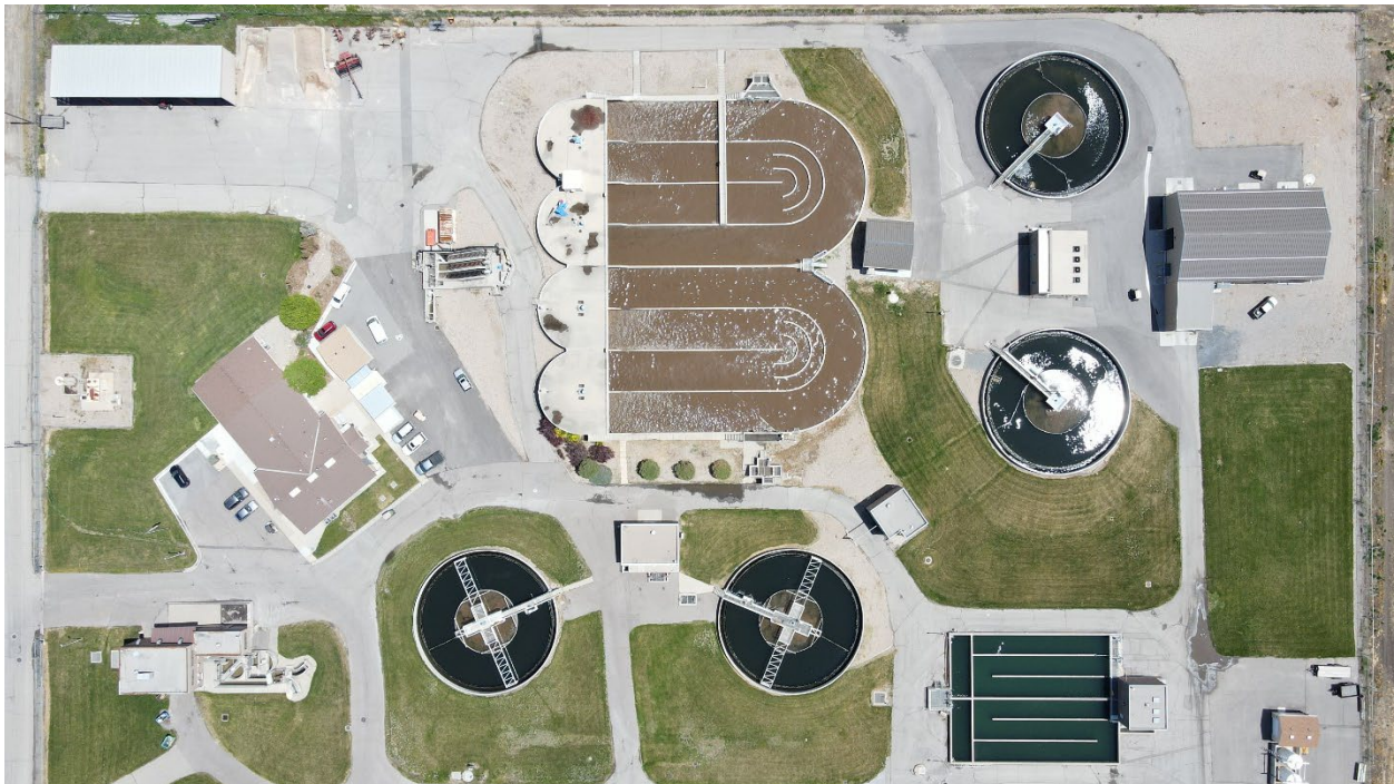
Figure 6: Oxidation Ditch Treatment Aerial
