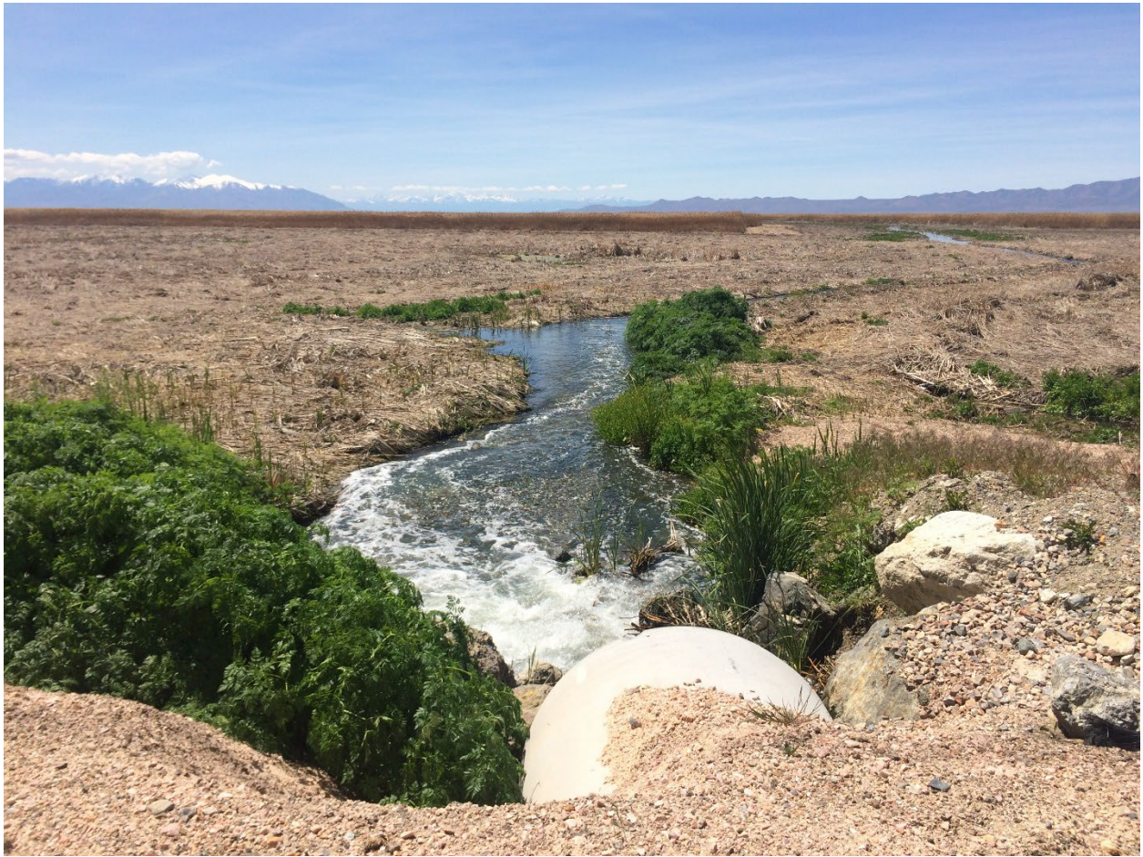
Figure 34: Central Davis Sewer District Outfall
