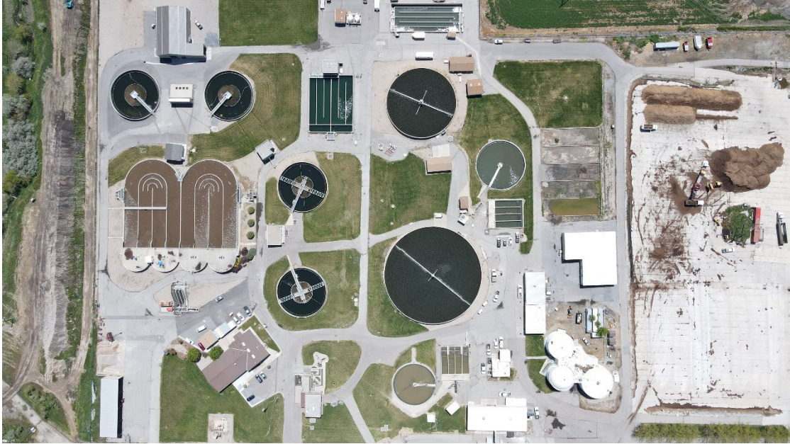
Figure 1: CSDS Treatment Plant
