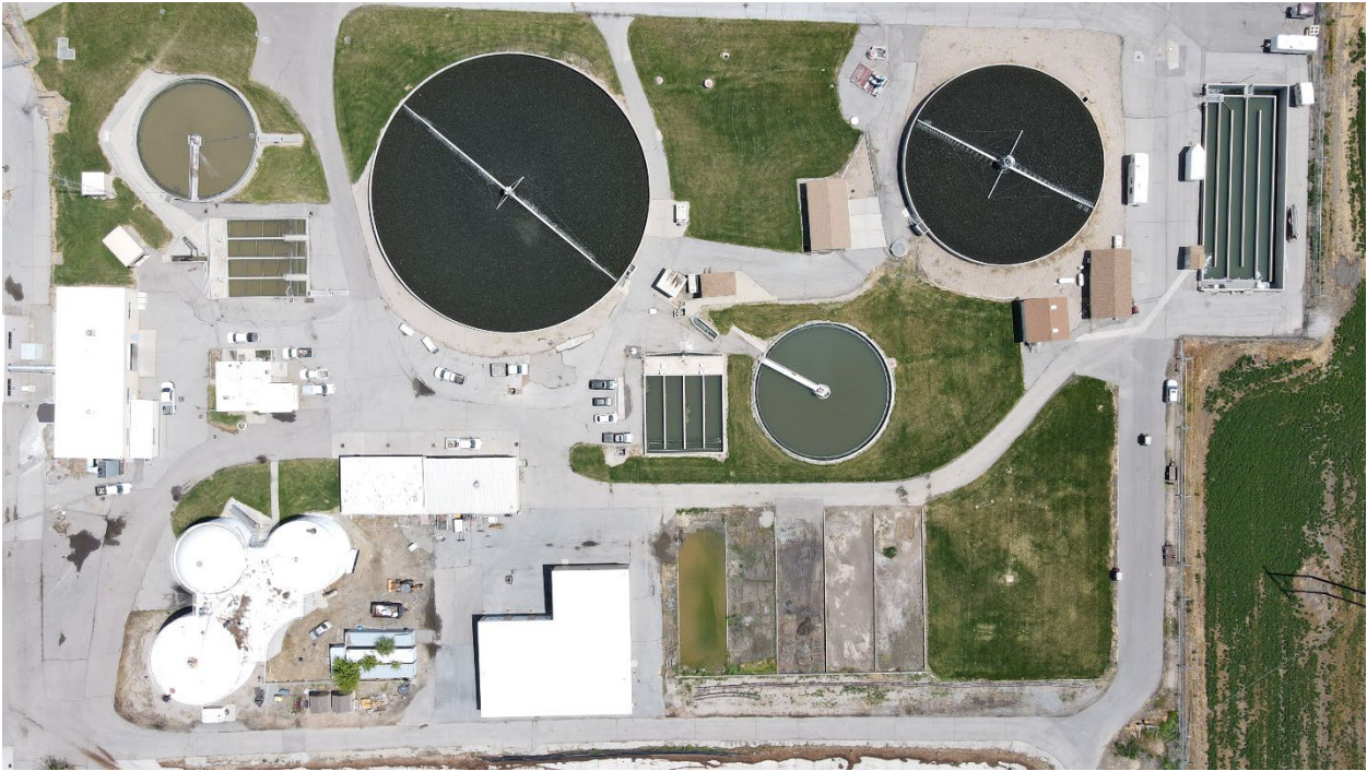
Figure 18: Trickling Filter System
