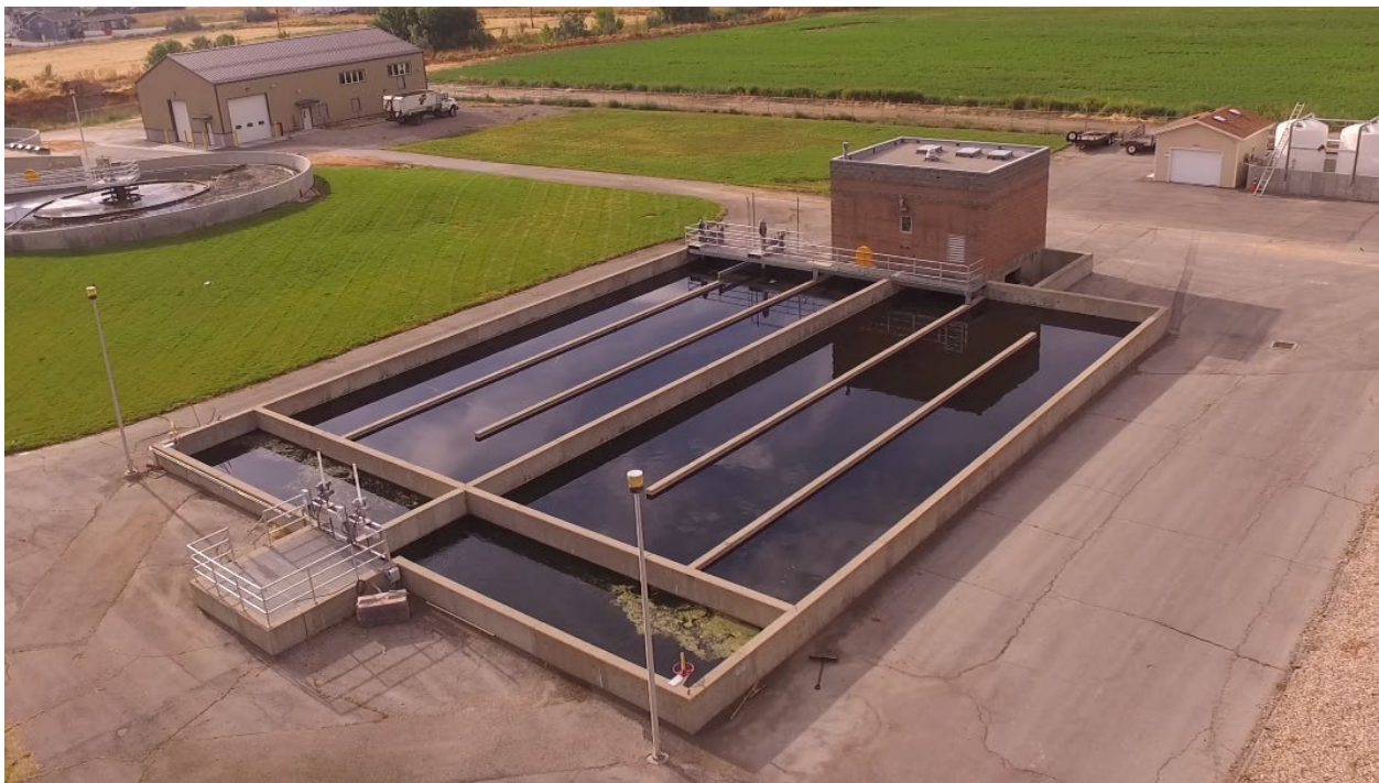
Figure 17: Chlorination Basin for Oxidation Treatment Train
