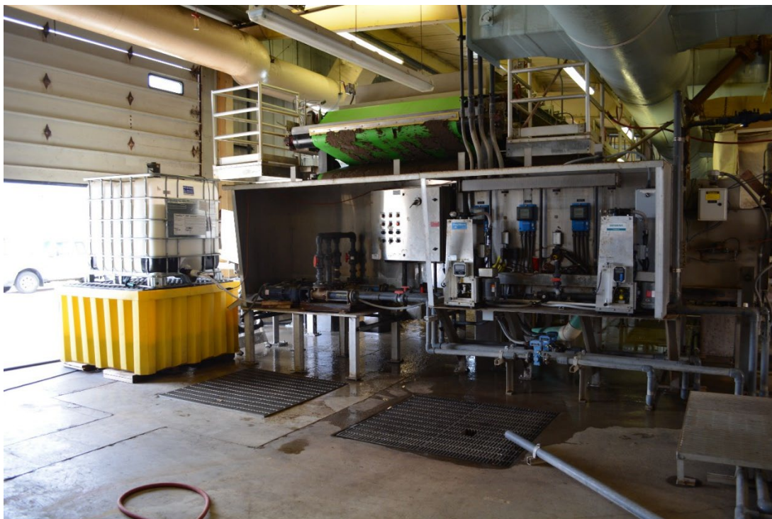
Figure 31: Belt Press and Polymer System
