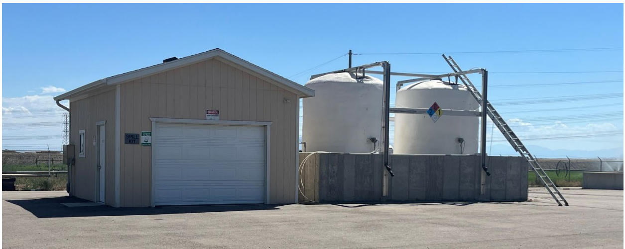
Figure 33: Sodium Hypochlorite Holding Tanks for Disinfection
