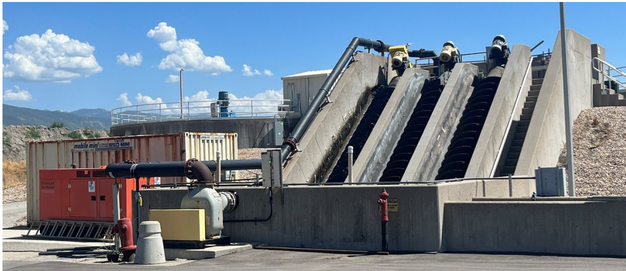
Figure 7: Screw Pump Station and Generators
