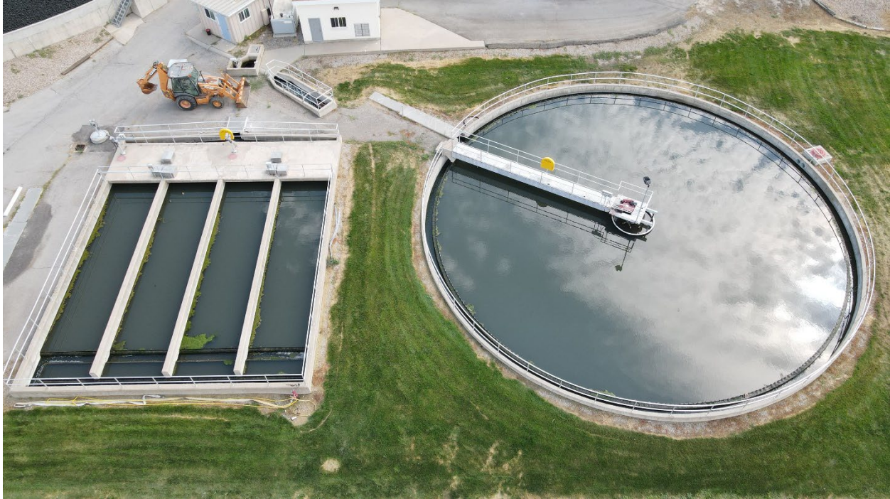
Figure 28: Secondary Clarifiers
