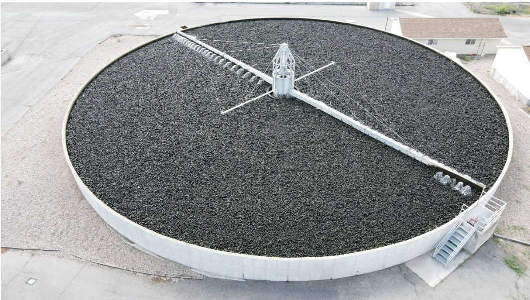
Figure 24: 2 nd Stage Trickling Filter
