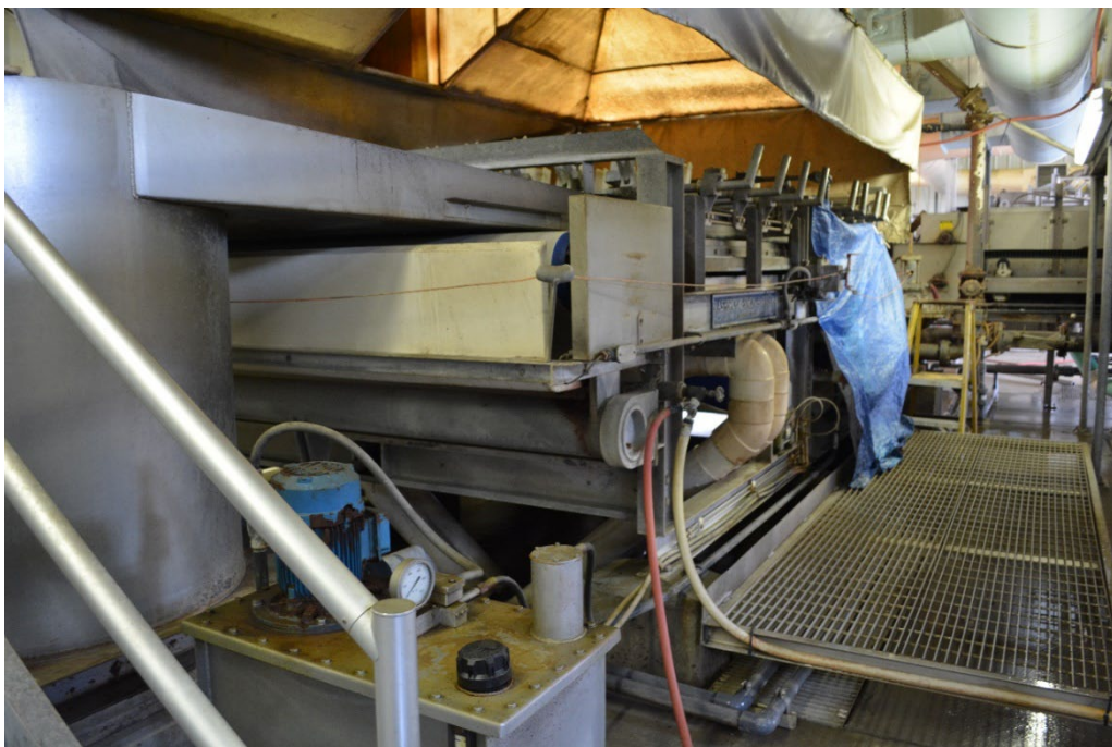
Figure 30: Gravity Thickener
