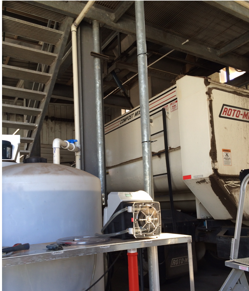
Blend Tank and Distribution Piping
