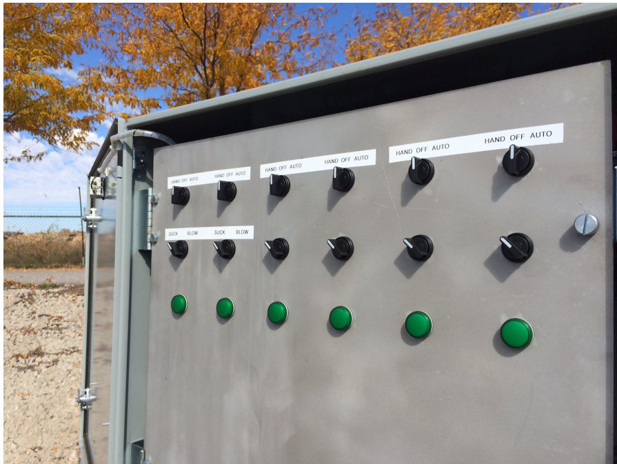
ASP Control Panel
