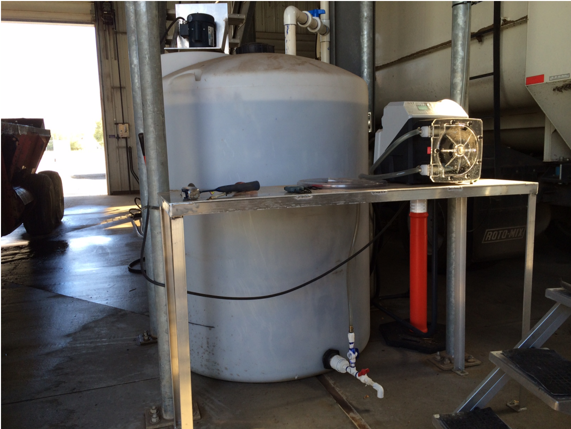
Blend Tank and Metering Pump
